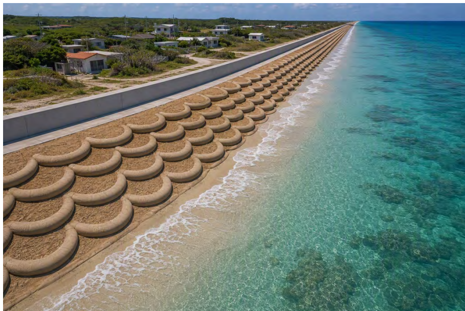
Fig. 16. Conceptual wave-dissipating stepped structure. The step is filled by coral gravel or small sand bags with the outer edge surrounded by sand tubes. Beachrock technology may be applied for both fill and sand tubes to enhance the stability. The permeable structure reduces wave reflection and run-up while promoting sediment accumulation and the formation of a gently sloping shoreline.
